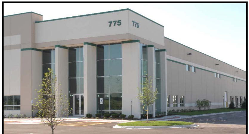
ProLogis Park 55, Building #4
